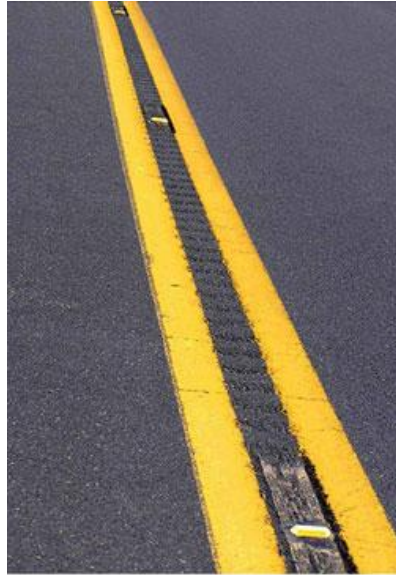
Recessed centerline pavement marking (Arizona DOT)
